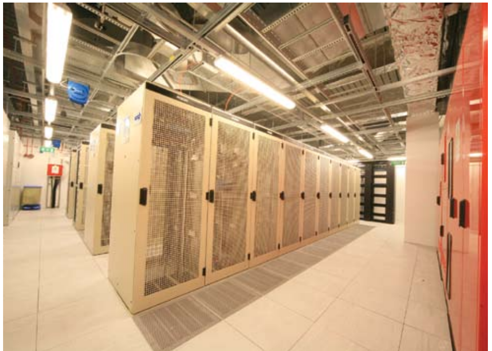
Kingspan access flooring in a UK data centre.
