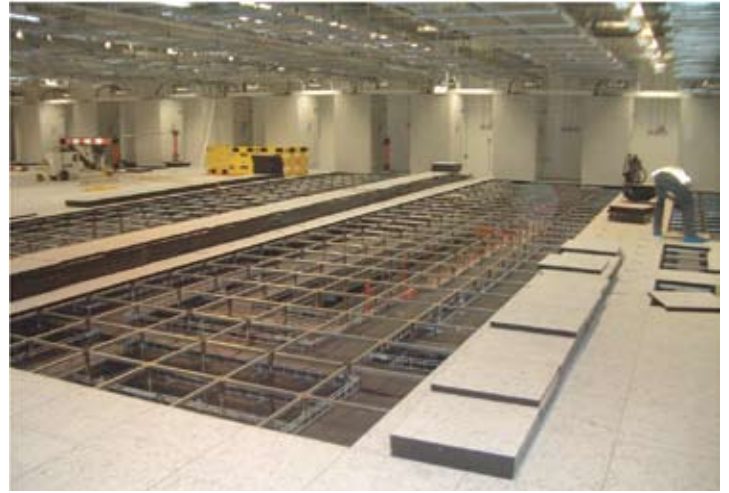
Kingspan access flooring being installed in a data centre in the UK. Clients have the option of a range of different finishes.
