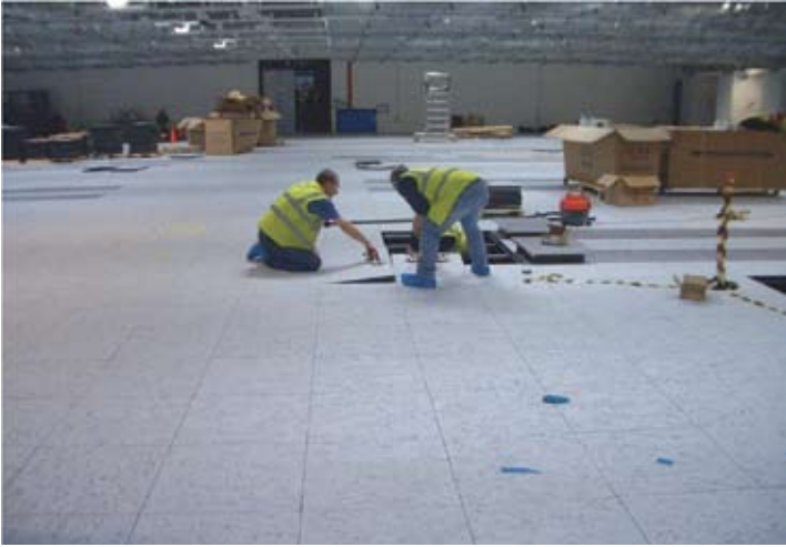
Kingspan access flooring being installed in a data centre in the UK. Clients have the option of a range of different finishes.
