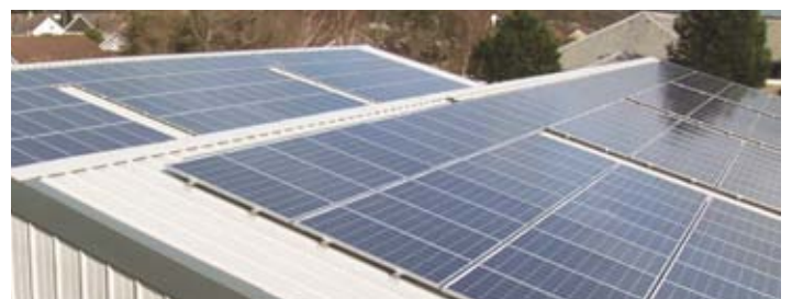
We have also installed 1,000 photovoltaic solar panels.
