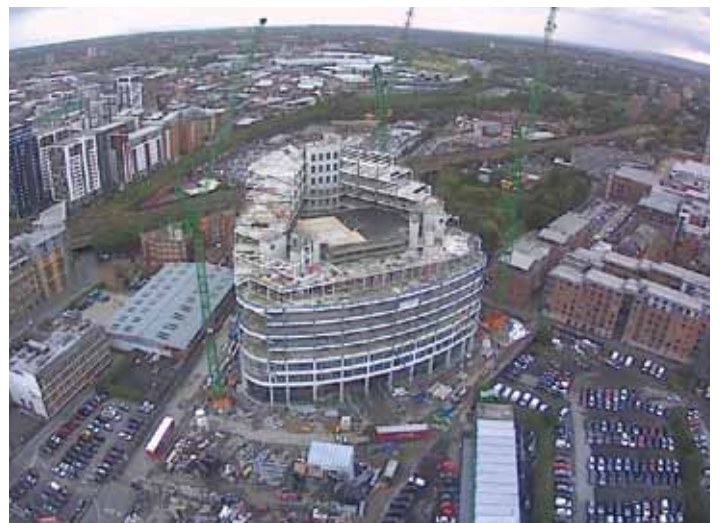
The new Co-operative head offices under construction.
